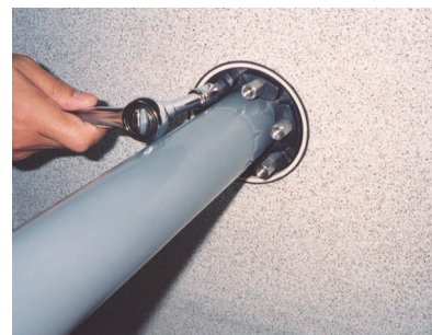
Socket wrench method (SSR) For medium and large diameters
