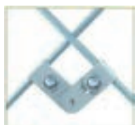
Example of anti-sway V-fitting installation
