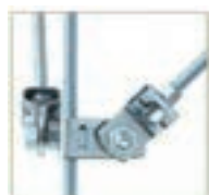
Example of anti-sway L-fitting installation
